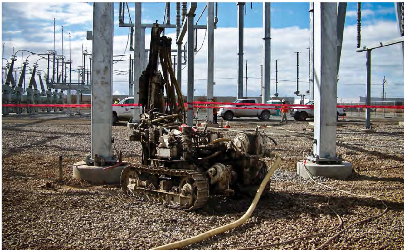
Populus Transmission Line, Salt Lake City, UT - Compaction Grouting to Improve Deep Foundation Capacity
